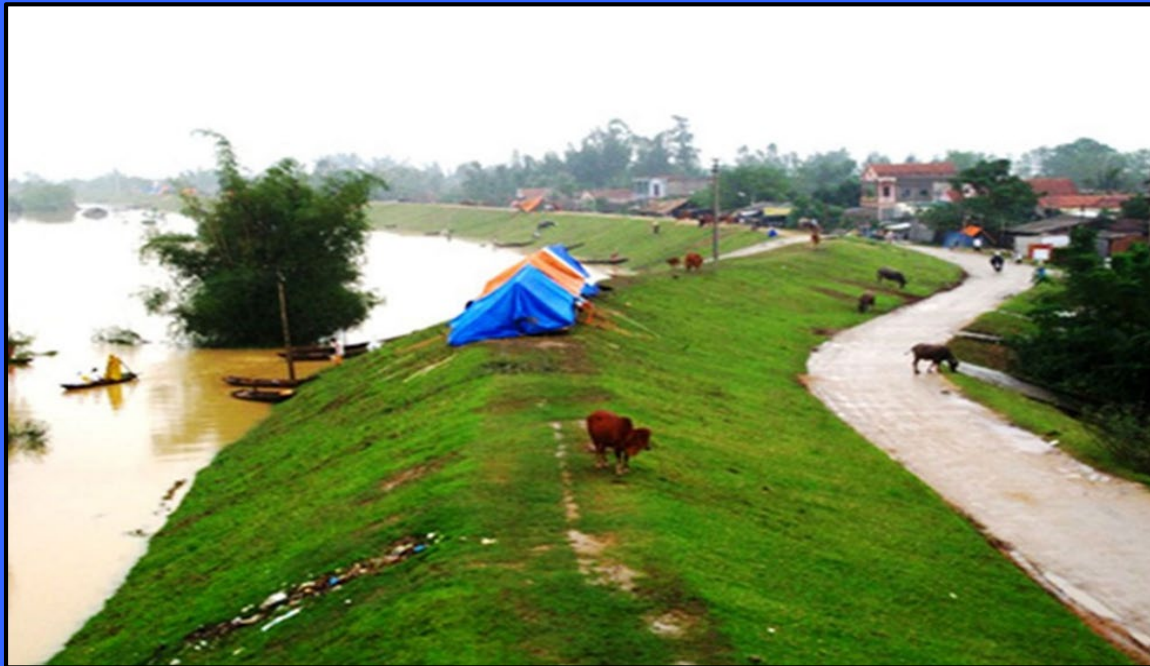
View of the dam along the Red River in Hanoi
