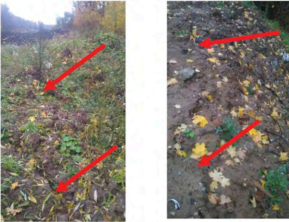
Figure 2. Cracks on the edge of the embankment.
